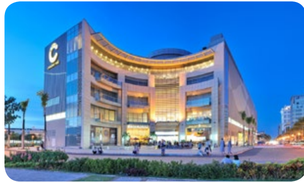
Crescent Shopping Mall - HCMC
