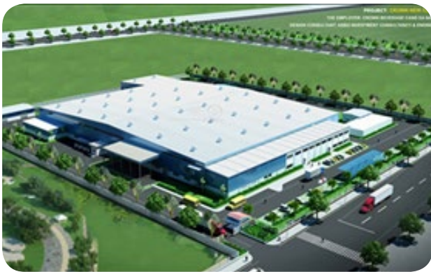
Crown New Can Project - Da Nang
