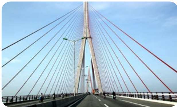
Can Tho Bridge Project
